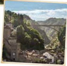
Galtertal bridge, Fribourg Region
